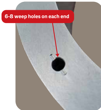
Fig. 1: Weep hole marked with a line
